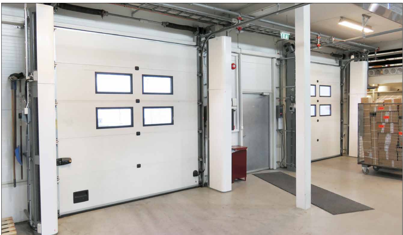
Vertical mounted Pamir 5000 with a vertical kit to allow two units to be installed on top of each other.
